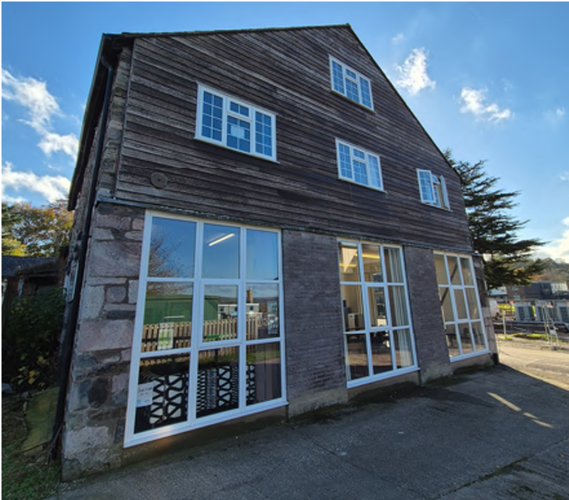
Figure 1: View of Gable Elevation
